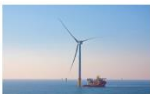
SSE, Equinor notch first power at Dogger Bank 9 OCTOBER 2023
